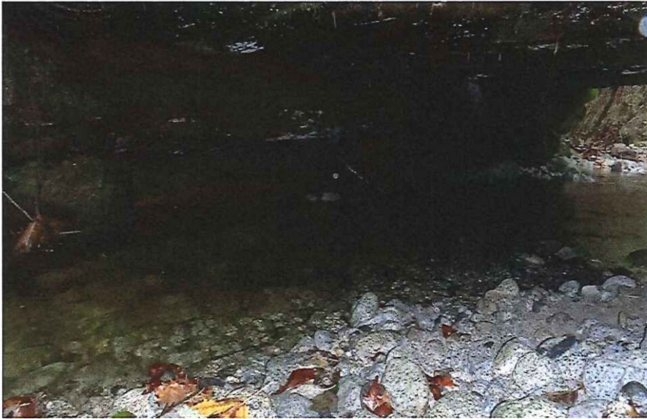
CK2331 Left Abutment
