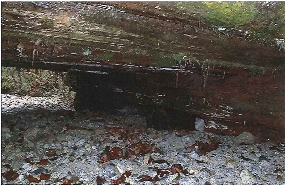
CK2331 Right Abutment
